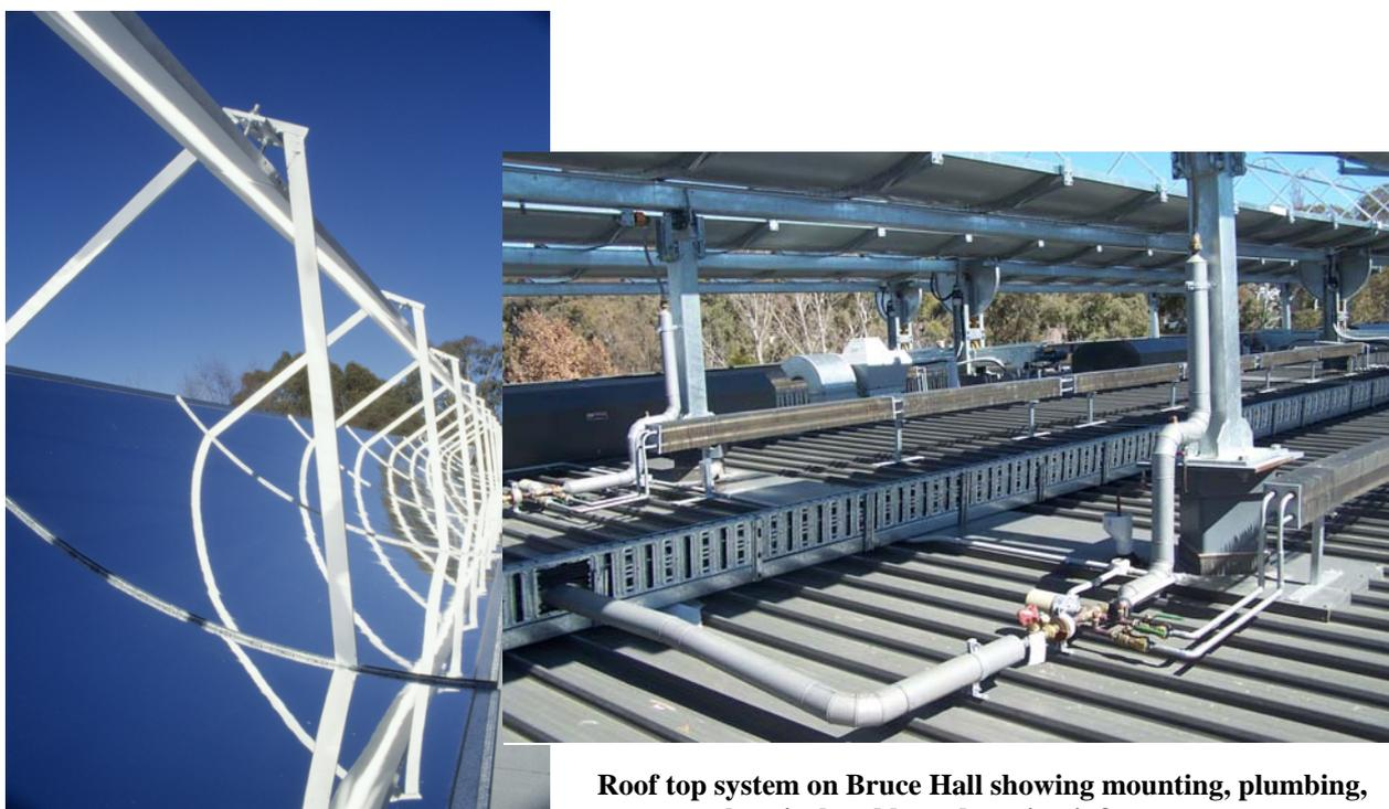
**Roof top system on Bruce Hall showing mounting, plumbing, electrical and heat dumping infrastructure**
